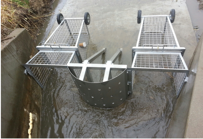
An installed DLT 400 GPT and DLT 400 diffuser
