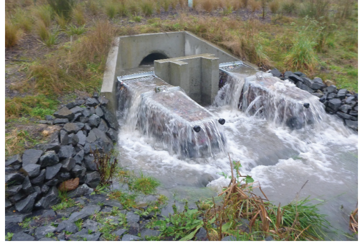
An installed DLT 400 system intentionally not maintained (100% filled with gross pollutants) demonstrating both retention of gross pollutants and SW flow and aeration during a 1 in 5 year event.
